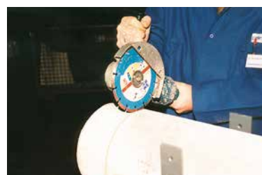
Cutting to length using a large angle grinder
